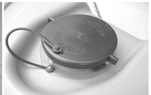
3" cap with strap attached--top of tank
